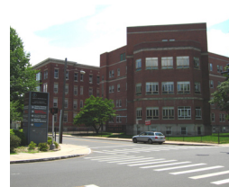
St. Francis Hospital
