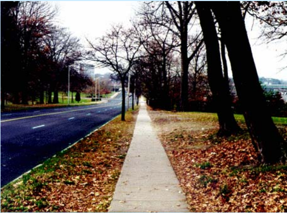
Concrete sidewalk on Park Street
