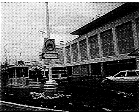
Parking is located under the supermarket.
