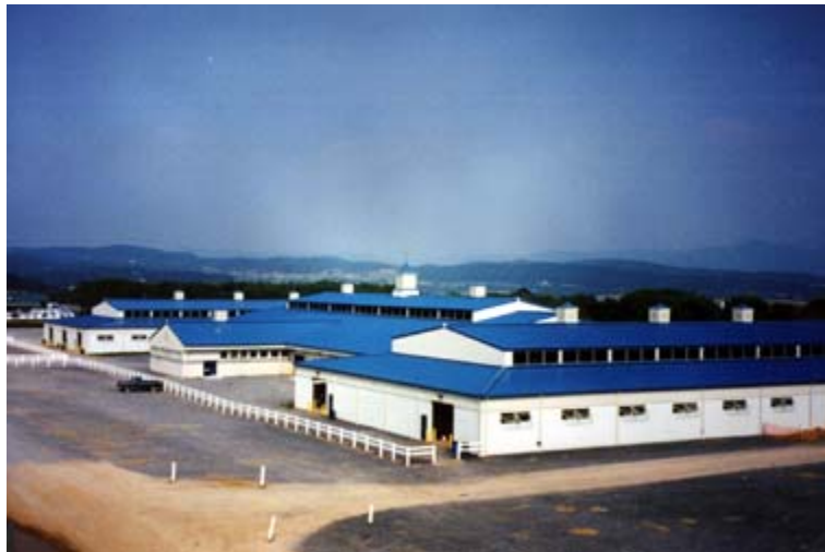
Figure 5 East Complex Barns of the Virginia Horse Center
