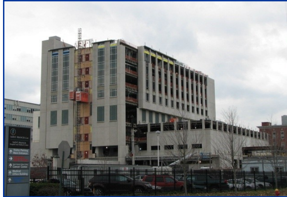
St Francis Hospital Surgical Tower
