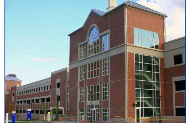
Aetna Expansion- Sigourney Street Garage
