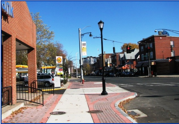
Park Street Streetscape
