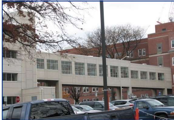
St Francis Hospital Expansion
