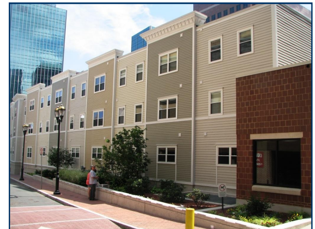
These townhouses are part of the 120-unit 18 Temple Street student complex
