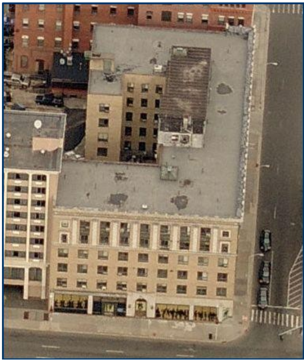
410 Asylum Street is being converted into apartments
