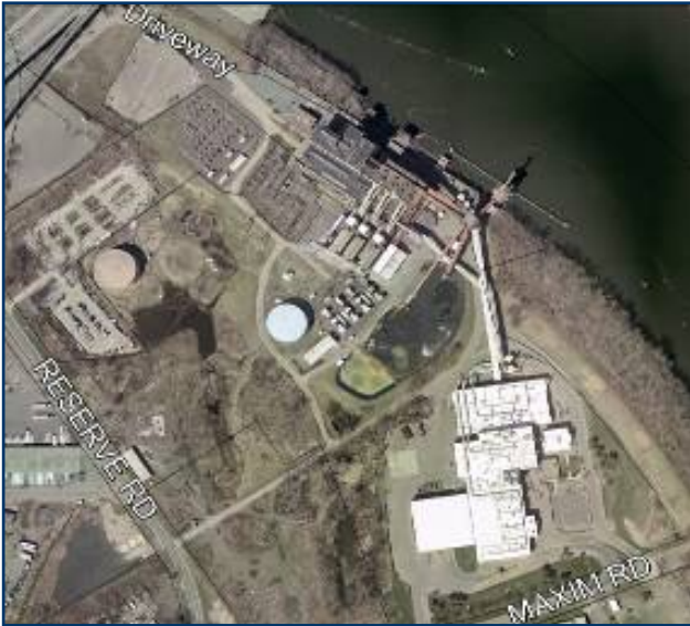
Aerial View of CRRRA's Mid-Connecticut Facility
