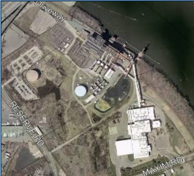
Aerial View of CRRRA's Mid-Connecticut Facility
