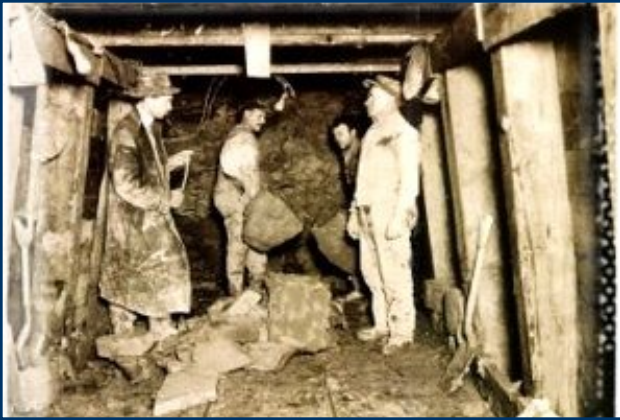
Construction of Hartford's sewer system began in 1929
