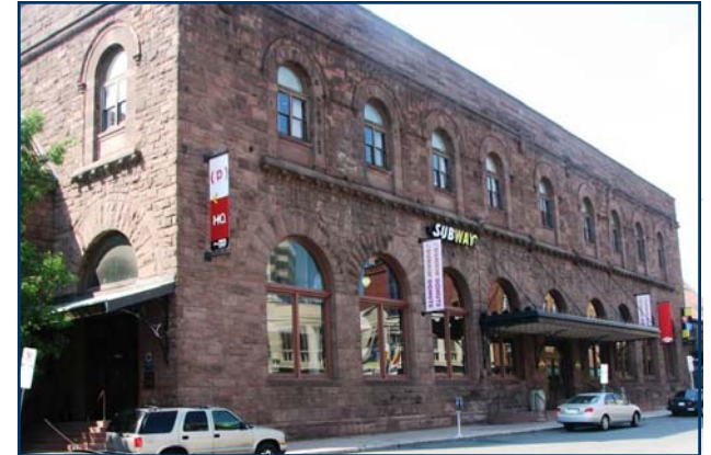
Union Station will become a multi-modal transit center
