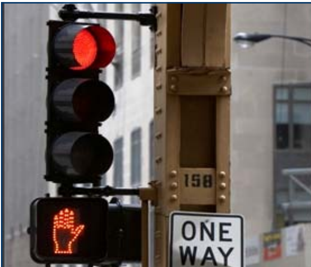
Replacing Hartford's traffic signal and street lights with LEDs will save energy and money.
