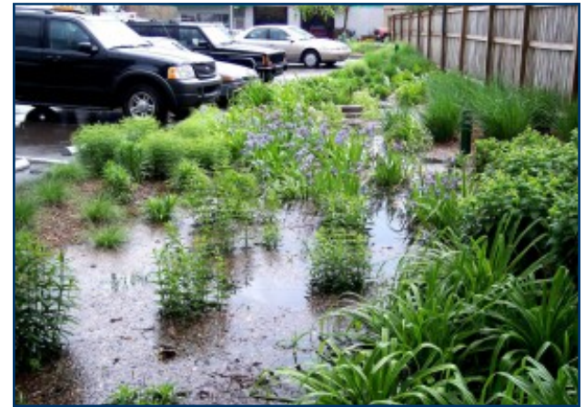
Rain gardens, or bio-retention basins, reduce stormwater runoff.
