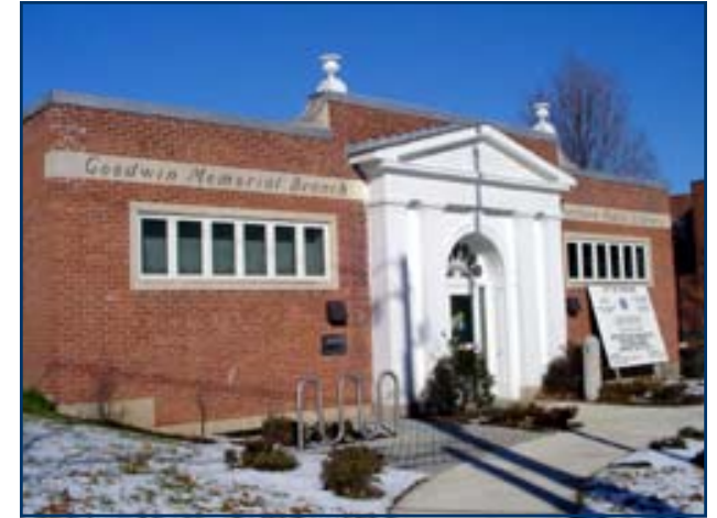
Goodwin Memorial Library has installed a solar photovoltaic system through the CT Clean Energy Options program.
