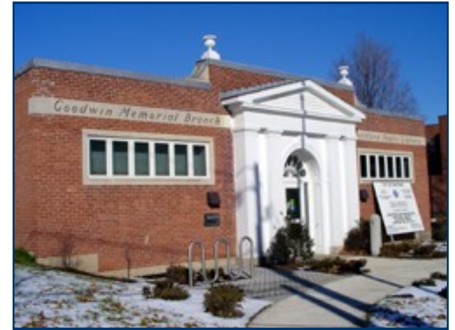
Goodwin Memorial Library has installed a solar photovoltaic system through the CT Clean Energy Options program.
