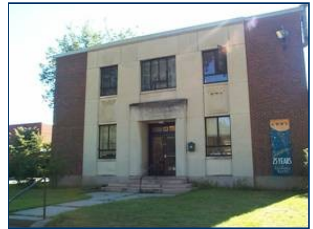
Recovery House, Northeast
