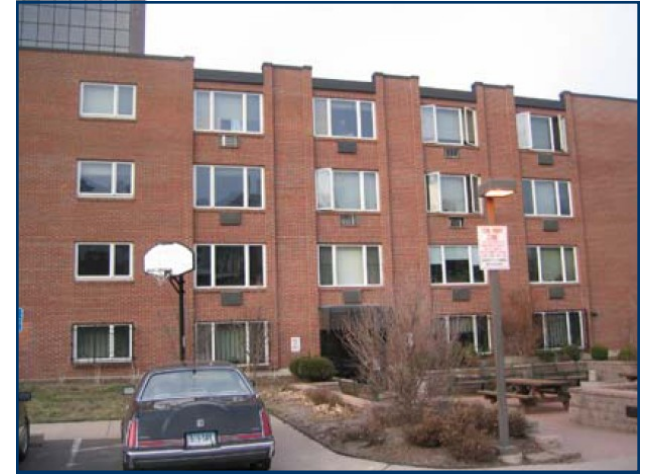
Hudson View Commons Supportive Housing, South Green
