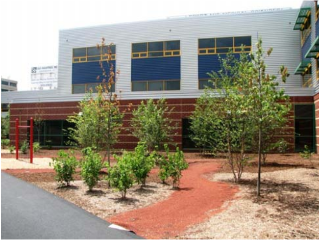
Pervious ground covering at the Sports & Medical Sciences Magnet School
