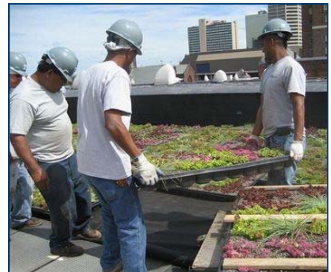
Installation of a Green Roof at the Betty Ruth and Milton B. Hollander Foundation Center
