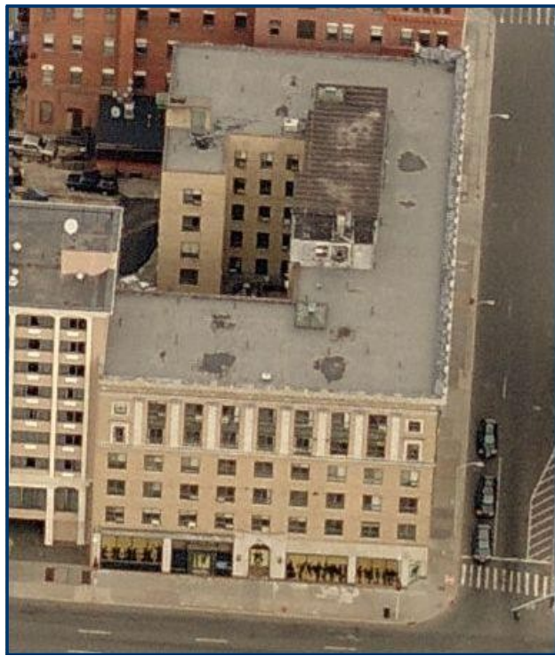
410 Asylum Street is being converted into apartments
