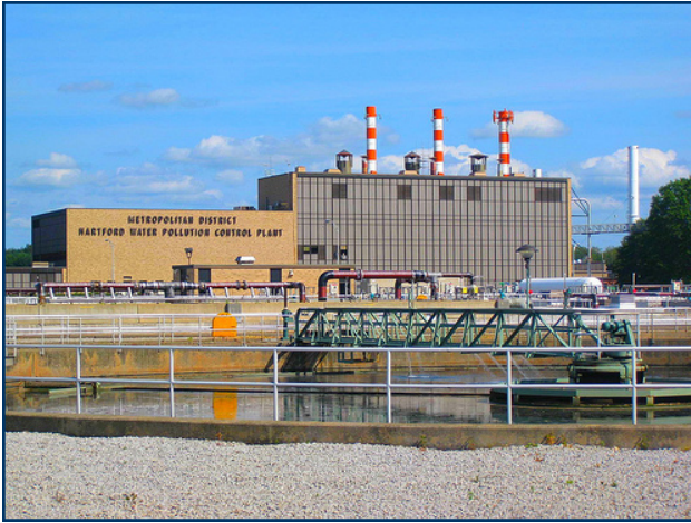
The MDC water treatment facility
