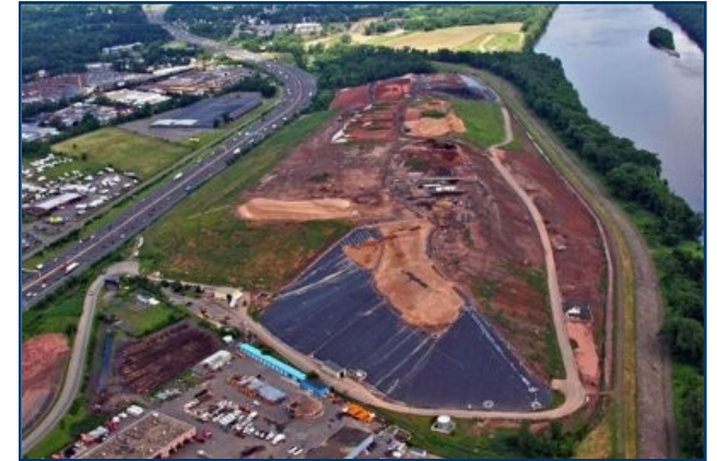
The Hartford Landfill is in the process of being capped.
