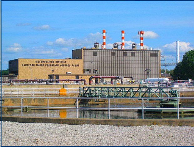
The MDC water treatment facility
