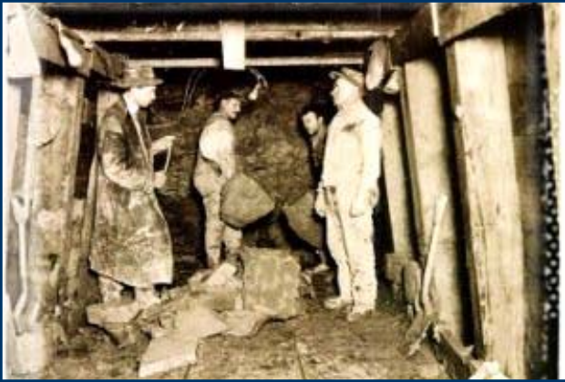
Construction of Hartford’s sewer system began in 1929
