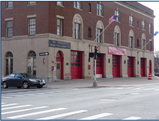
Fire Dept. Headquarters Pearl St.
