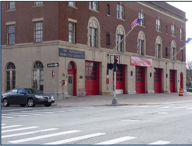
Fire Dept. Headquarters Pearl St.
