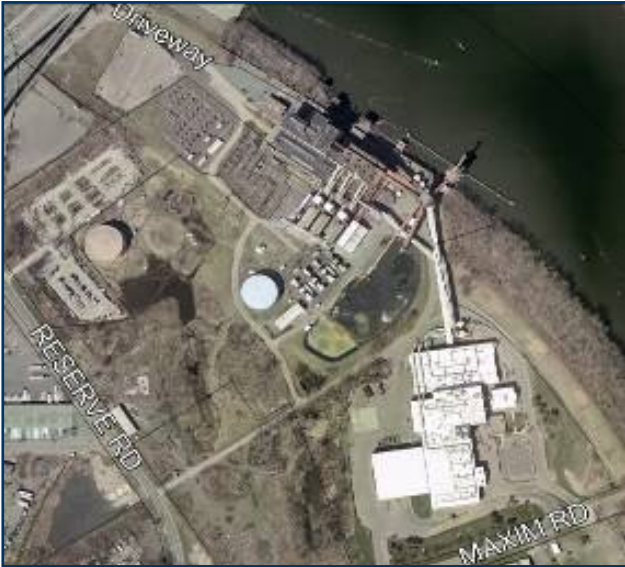
Aerial View of CRRRA's Mid-Connecticut Facility
