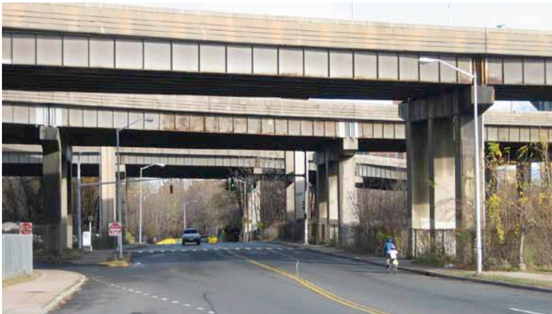
Capitol Avenue, near the Sisson Avenue interchange, passes below multiple highway ramps and the rail line, creating a sharply defined barrier between surrounding neighborhoods and downtown Hartford.
