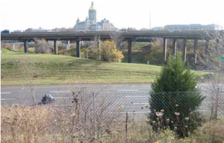
The Viaduct and its ramps divide the city—separating downtown and the Capitol from surrounding neighborhoods, and each other. Much valuable land is wasted.
