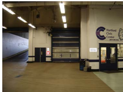
Roll up door from loading dock to marshalling area. Production trucks must be loaded and unloaded with ramps, which increases labor costs and time for loading and unloading equipment
