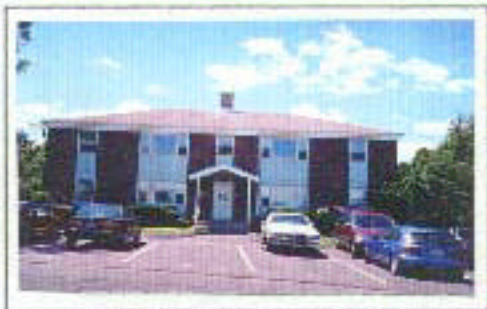
Parking in front of building non-descript facades
