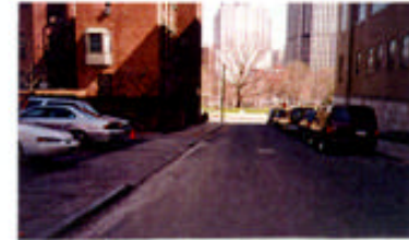
Large curb cuts reduce sidewalk safety
