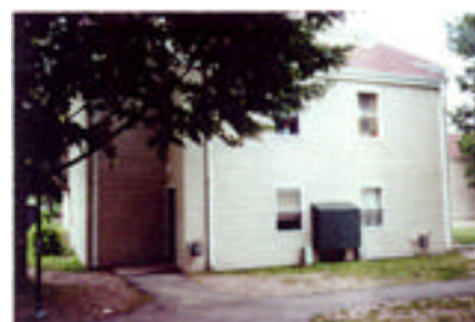
No defensible outdoor space (yard) makes it difficult to control who approaches the living unit
