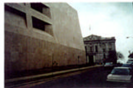
Blank facades reduce sidewalk safety
