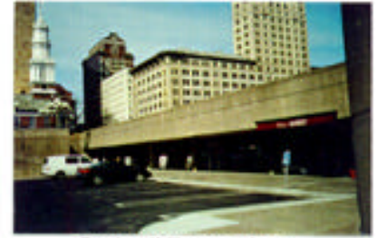
Bushnell Towers shop facing parking lot
