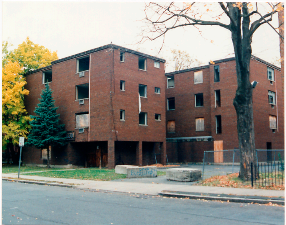
To the right is 54 Huntington, also scheduled for demolition.
