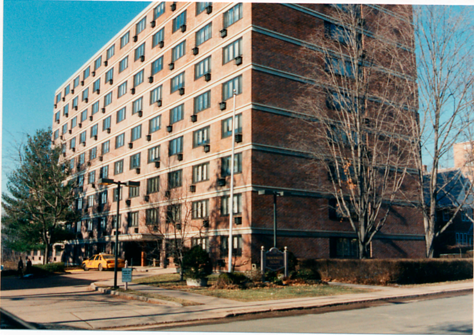
Pictured above is Immanuel House, a senior housing complex on Woodland Street.
