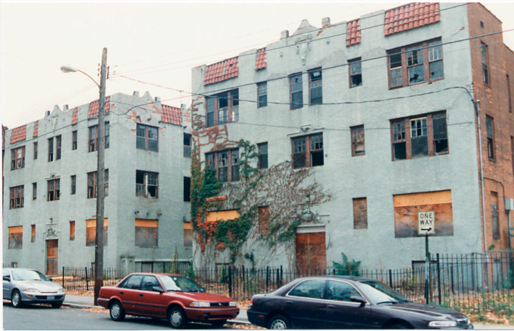
Pictured to the left is 3-11 Huntington, scheduled for demolition.
