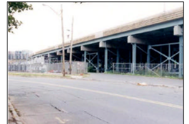
Northern Crossing of Van Dyke Avenue
