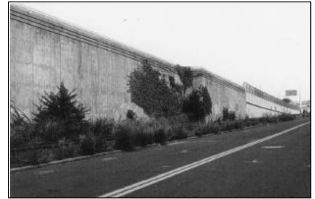
Van Dyke Avenue Existing Support Wall for I-91
