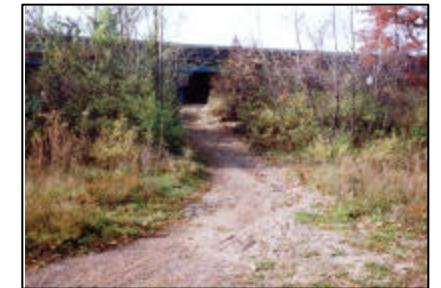
Existing Trail on the West side of the Dike
