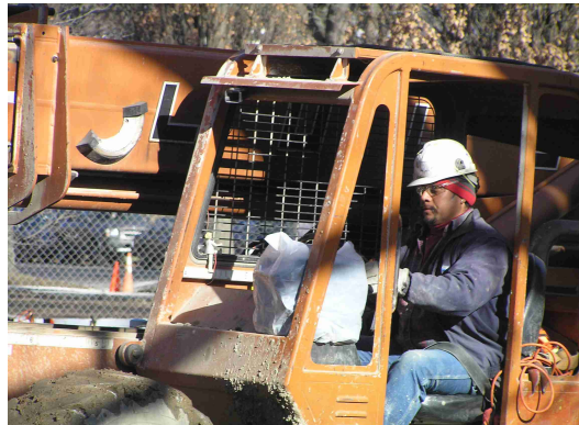
School construction means jobs!
